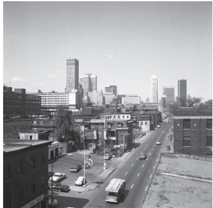
Figure 12. Looking east along rue Saint-Antoine from the roof of the Canadian Buttons Limited factory, 31 May 1967. Richmond Square is located midway up the street. Everything north of the street, or to the left, was demolished as part of highway construction. Everything to the south, or the right (except the Tynedale Centre in the foreground), was demolished as part of the urban renewal project. VM94-C1027-022, Archives de Montréal .
