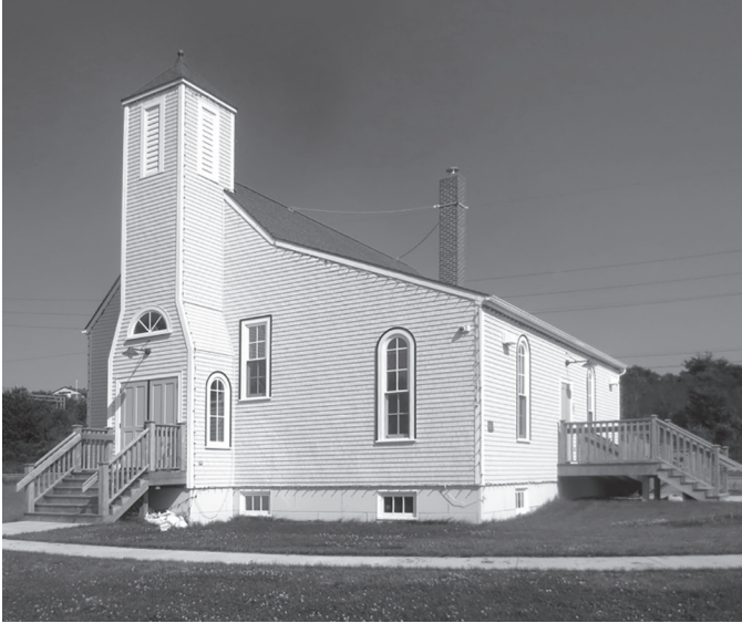
Figure 5. Rebuilt Africville Church. Photograph by V. Prouse.
