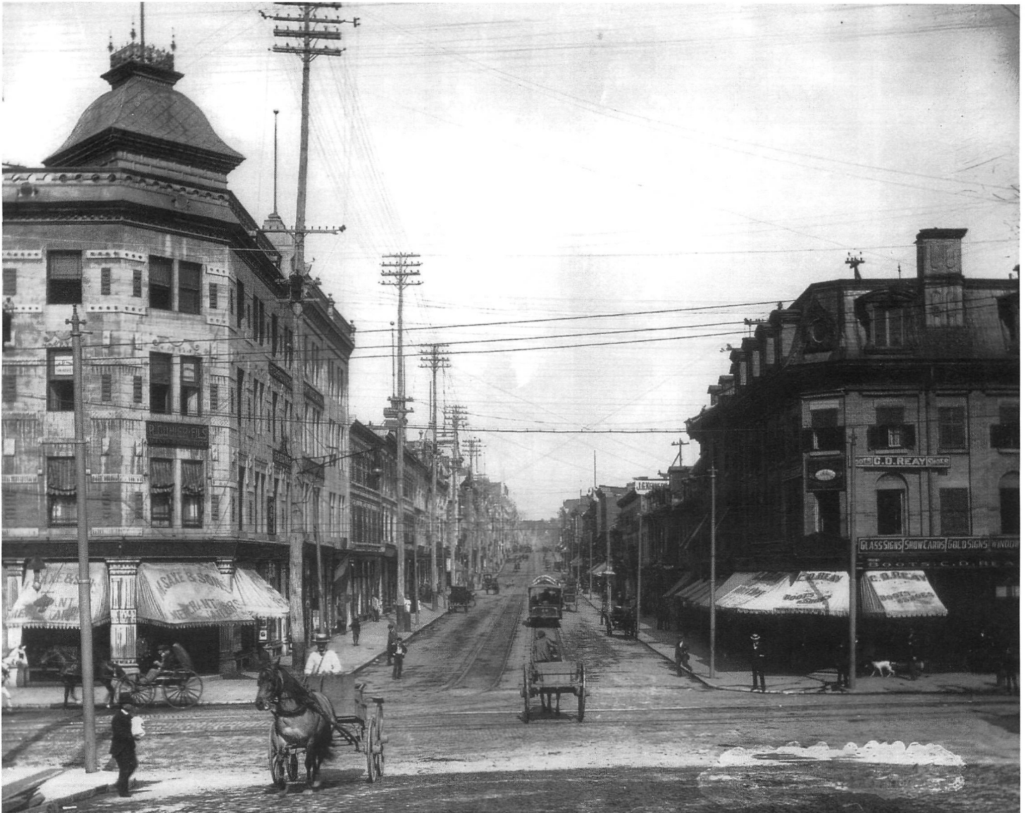
Figure 5: St Lawrence Street corner Craig Street, rebuilt after widening, circa 1892
