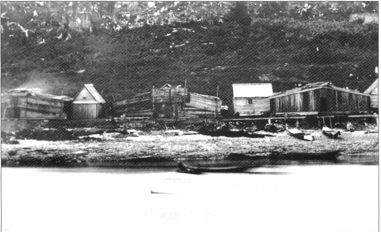
Figure 2: Detail of Figure 3 showing Native-style houses, each with small associated structures of distinctly European appearance, which may have been moved to the village at the time of the abandonment of Fort McLoughlin in 1843. The two plank houses on the left show horizontal removable siding. The one on the right shows more permanent fine vertical siding.
