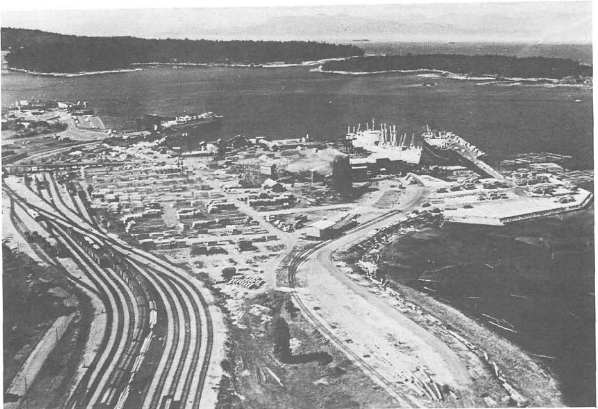
Photograph #5: Deepsea lumber assembly wharf and rail and motor vehicle ferry terminuses are the key to Nanaimo's post war expansion as a trans-shipment point and distribution centre. Most of the complex was built on mine waste fill, much of it from No. 1 mine which was located to the left of the curve in the tracks. Other coal mines were on Newcastle and Protection Islands across the harbour. (Victoria Press Limited photograph).
