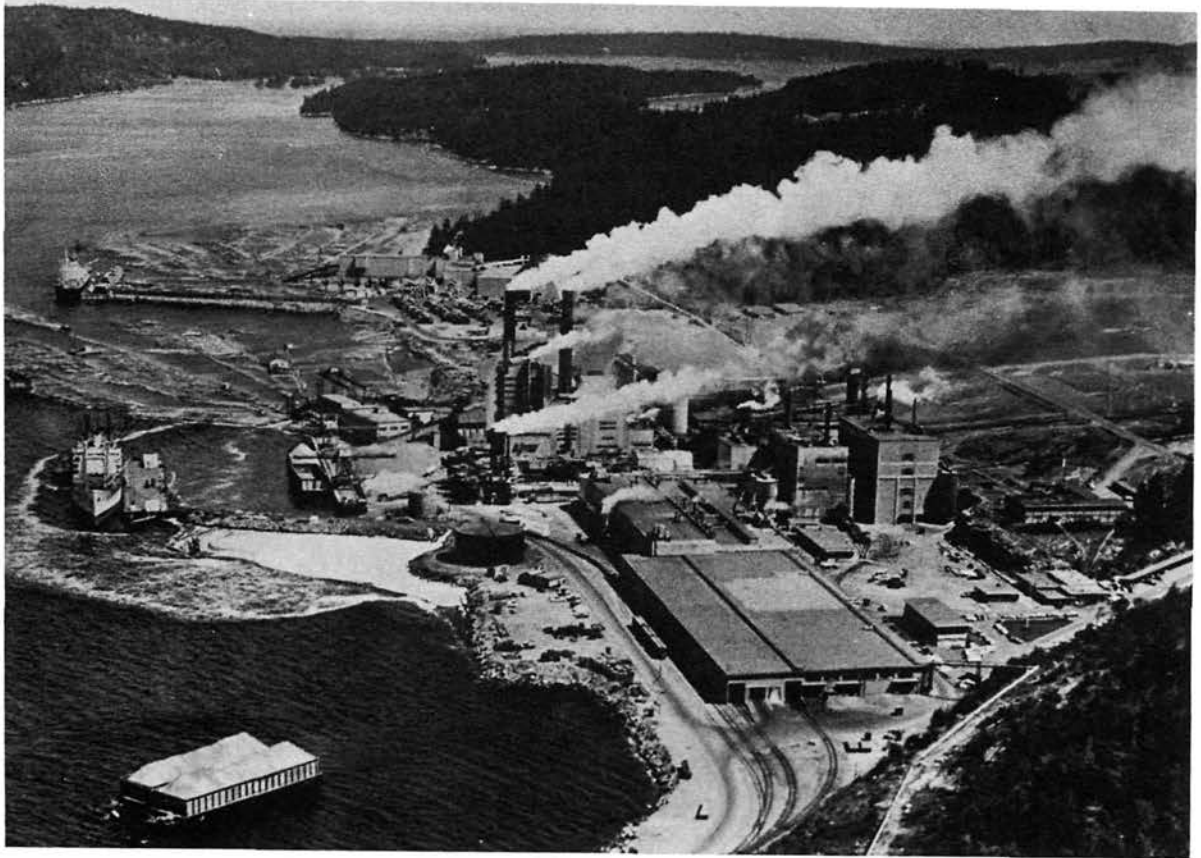
Photograph #4: Harmac, four miles southeast of Nanaimo, was built in 1949 by the H.R. MacMillan Export Company and is today part of MacMillan Bloedel Limited. The original pulp mill was rapidly expanded and it is now the region's single largest employer. About 1,100 people work in the mill and related operations. (Victoria Press Limited photograph).
