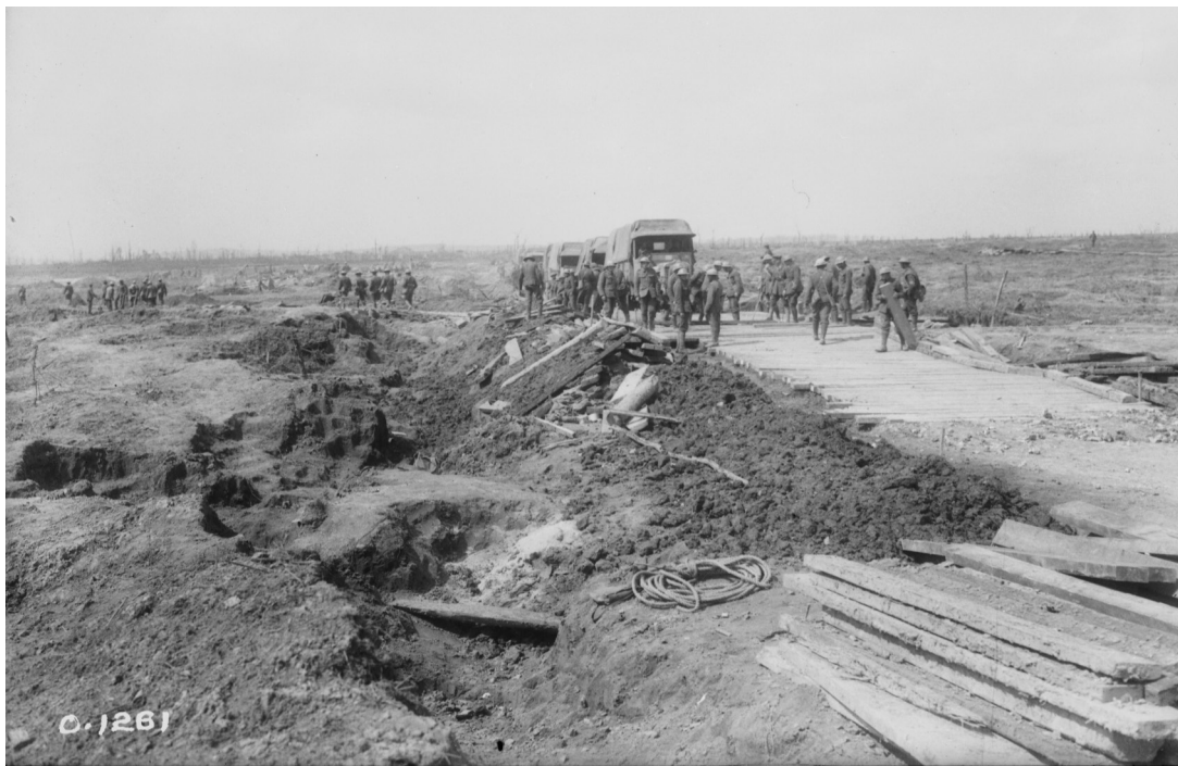
Figure 5. Laying a road over the crest of Vimy Ridge. April, 1917. Source: PA-001226, box number: 83,7435, 15, O-1261, Library and Archives Canada.
