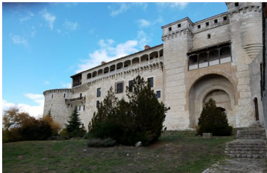
Figure 2. The gallery on the southern wall of the castle, towards the gardens. Castle of the dukes of Albuquerque, Cuéllar (Segovia).
