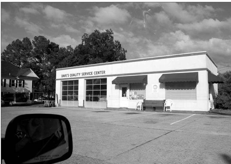
Fig. 15 Gasoline station with garage for vehicle maintenance, a common feature ca. 1930 through the 1960s. This particular station was built in the 1950s as evidenced by its oblong-box architecture with straight edges. It is currently an independent garage and no longer operates as a gasoline station. (Photo by authors.)
