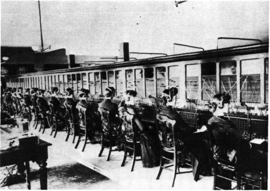
First multiple switchboard in Montreal installed in the British Empire Assurance Company Building, April 1886. At that period, all the operating labour force in big exchanges was constituted of women. (Photo #3109 Courtesy of Bell Canada Telephone Historical Collection)
