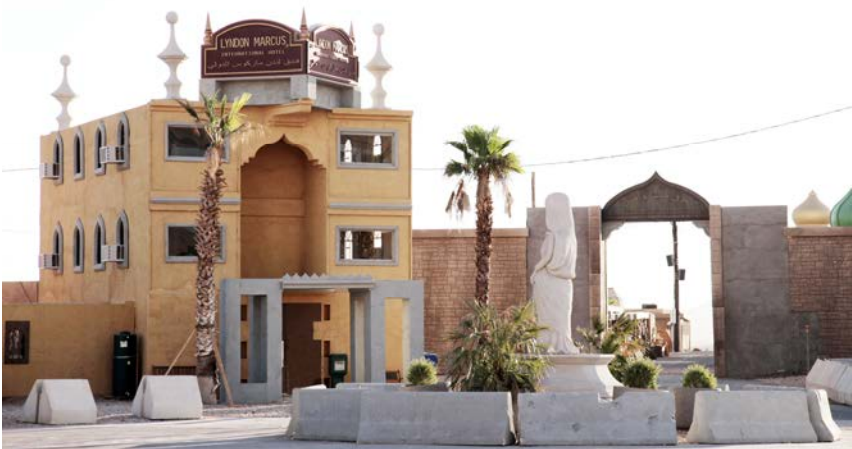
Fig. 2. The hotel where journalists are staying in Medina Wasl at Fort Irwin National Training Centre is, alongside the mosque, the tallest and most richly decorated building in the village. © Emanuel Licha
