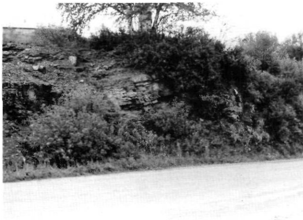
FIGURE 2. Faulted limestone on the Lindsay Formation, south side of Sim Street, Little Current.
