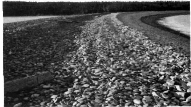
FIGURE 8. Ground view looking southwest along the barrier crest, north line, Fancys Point, 17 June 1991.
