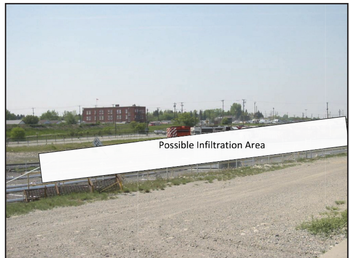
Figure 2. Possible location for discharge of treated groundwater to the aquifer (note the coarse-grained material in foreground).
