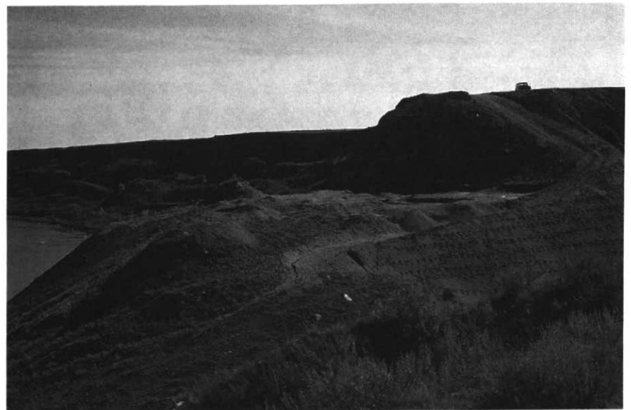
Figure 16 Excavation at Mitchell Bluff, South Saskatchewan River Valley, Medicine Hat, Alberta. Excavated face is topped by till and stratified sands and minor gravels below are of Mid-Wisconsinan or Sangamonian age. Sandy soil has been bulldozed to the right and as there are bones within the sands, the slope has been walked to search for them. The pattern of footprints illustrates the procedure described in the text.
