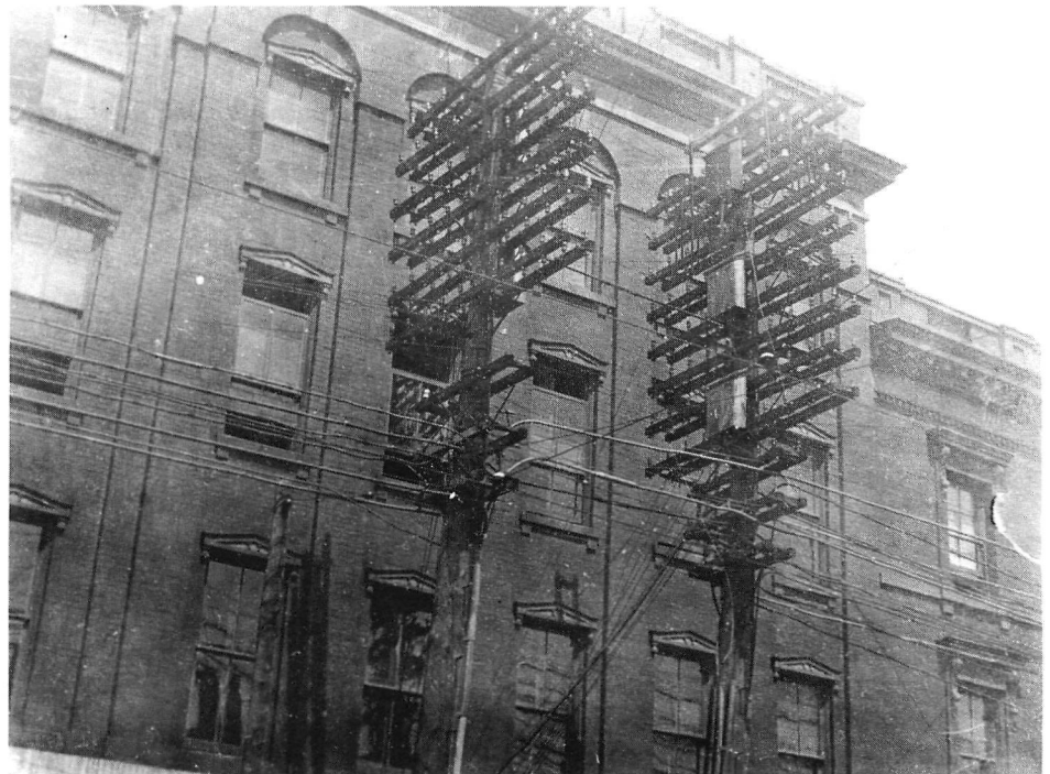
Figure 2: The Wired City. Poles in front of Bell Canada central office, Kingston, Ontario, 1903.
