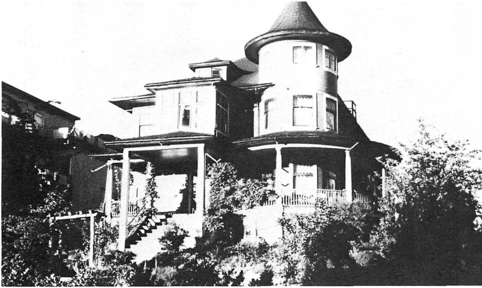
House in Broughton District, Vancouver
