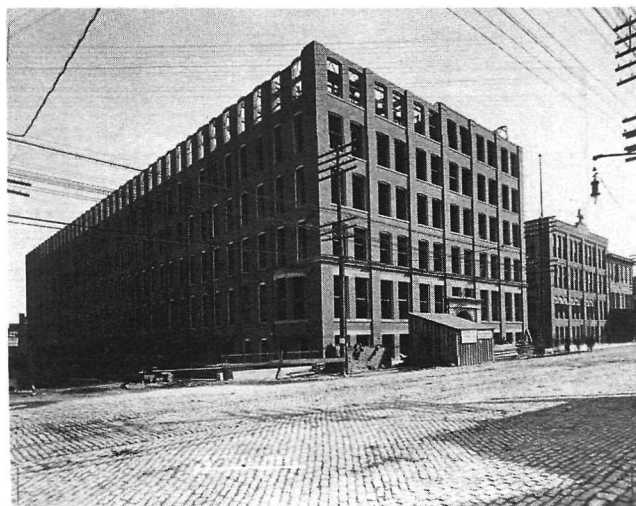
FIGURE 2. John Deere Plow Company Warehouses, St. Louis, Missouri. Architect – Eckerman. October 16, 1903
