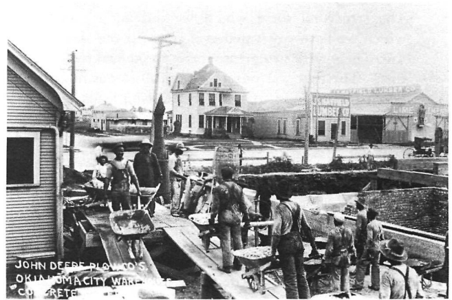
FIGURE 8. Concrete Mixing, John Deere Warehouse, Oklahoma City
