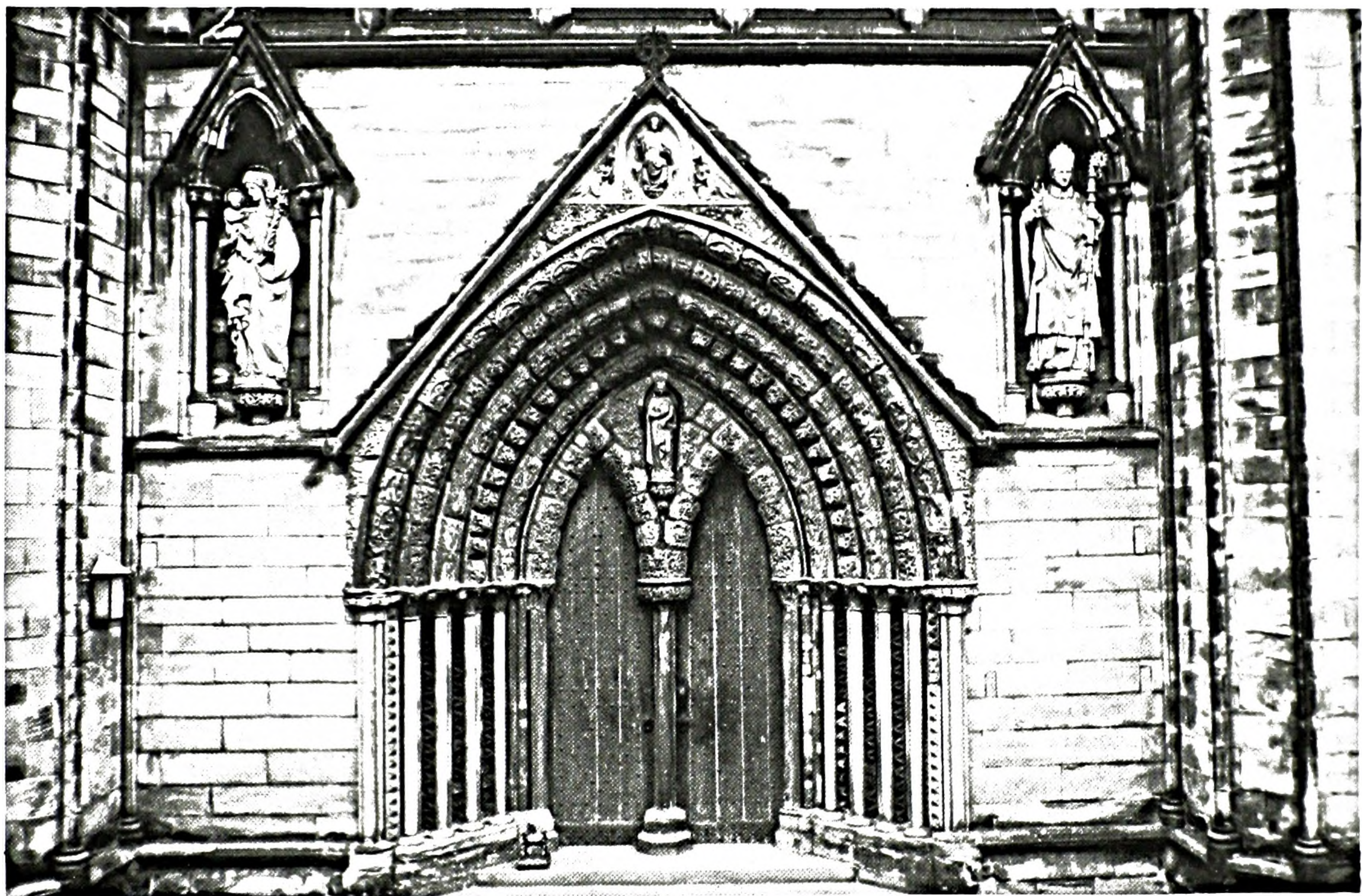
FIGURE 1. Lichfield Cathedral, north transept doorway (By courtesy, the Dean and Chapter of Lichfield Cathedral).
