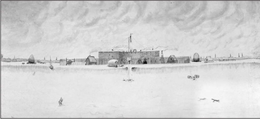
Figure 3: A south-east view of Albany Factory, William Richards, (c1800) HBCA.
