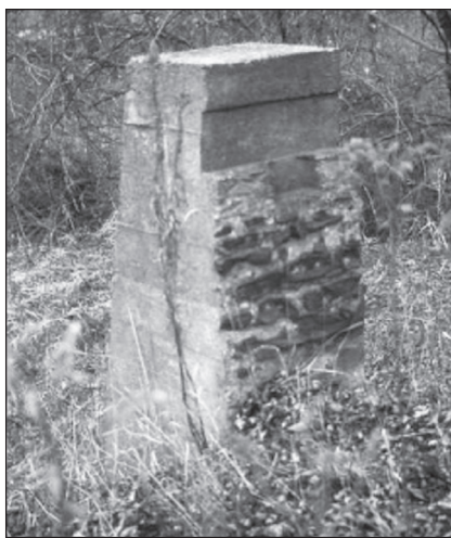
FIGURE 11. This pillar of poured concrete bears the imprint of a beam and foundation stones in the Silverthorn Mill, torn down in 1954. It is a memorial to the founding of this industrial village more than 160 years ago, and was still standing in 2012. (Author photo)
