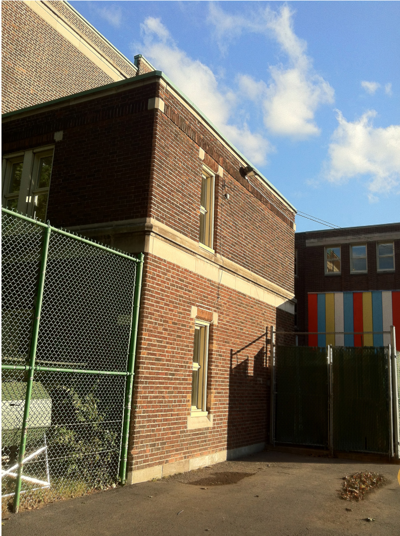
FIGURE 2. Guy Drummond yard (north view)
