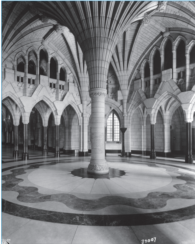
FIG. 1. CONFEDERATION HALL, WITH VIEW OF CENTRAL COLUMN AND HALL OF HONOUR, CENTRE BLOCK, PARLIAMENT HILL, OTTAWA, ON, 1920, PHOTOGRAPHED IN 1936. LIBRARY AND ARCHIVES CANADA / CANADIAN NATIONAL RAILWAY COMPANY FONDS / E010861885.
