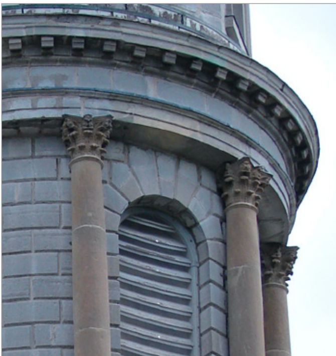
FIG. 48. ST. GEORGE'S CHURCH, BELFRY, 1842; DETAIL OF CORINTHIAN COLUMNS AND ENTABLATURE. | PHOTO: PAUL CHRISTIANSON, JULY 2022.
