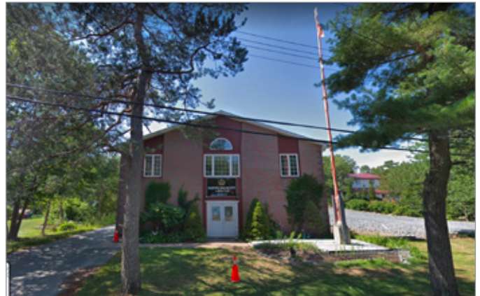
FIG. 30. THE GURDWARA OF THE MARITIME SIKH SOCIETY (1978), 10 PARKHILL ROAD, HALIFAX, NS: [HTTPS://WWW.GOOGLE.CA/MAPS/@44.6243341,-63.6006573,3A,75Y,309H,100.82T/DATA=!3M6!1E!13M4!1STMLUGSIZTGCK7RNKYFW4HQ!2E0!7!16384!8!8192?HL=EN]. | GOOGLE MAPS.
