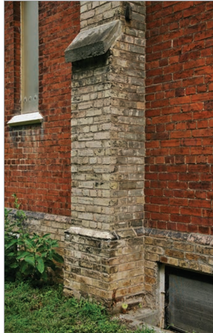
FIG. 24. MCNAB, CHRIST CHURCH ANGLICAN, BUTTRESS DETAIL. | MALCOLM THURLBY.
