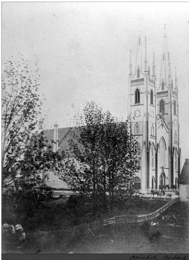
FIG. 1. VIEW OF THE THIRD CHURCH OF THE PARISH OF LA NATIVITÉ DE NOTRE-DAME, BEAUPORT, C. 1885. CHARLES BAILLAIRGÉ, ARCHITECT (BUILT 1849-1852). | UNKNOWN PHOTOGRAPHER. ARCHIVES DE LA VILLE DE QUÉBEC, FONDS MICHEL BÉDARD, P110-200-2-2-N083233.
