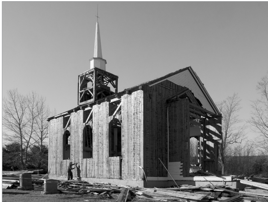
FIG. 9. ALL SAINTS, GRANVILLE CENTRE, NS, DURING DEMOLITION. | PETER COFFMAN.
