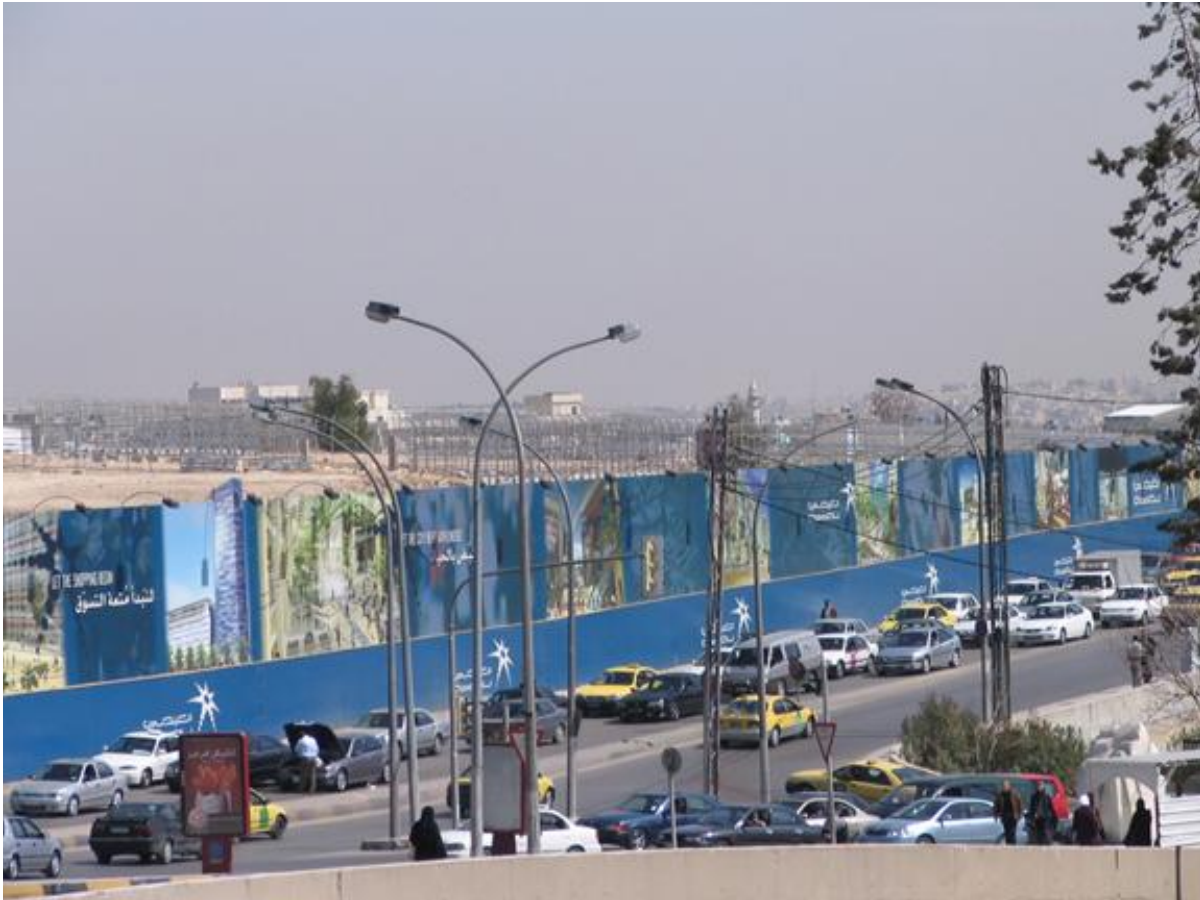
Fig. 1 - A stretch of billboards around the Abdali site during its early stages of construction some 4 years ago. (Photo Credit: Rami Daher)
