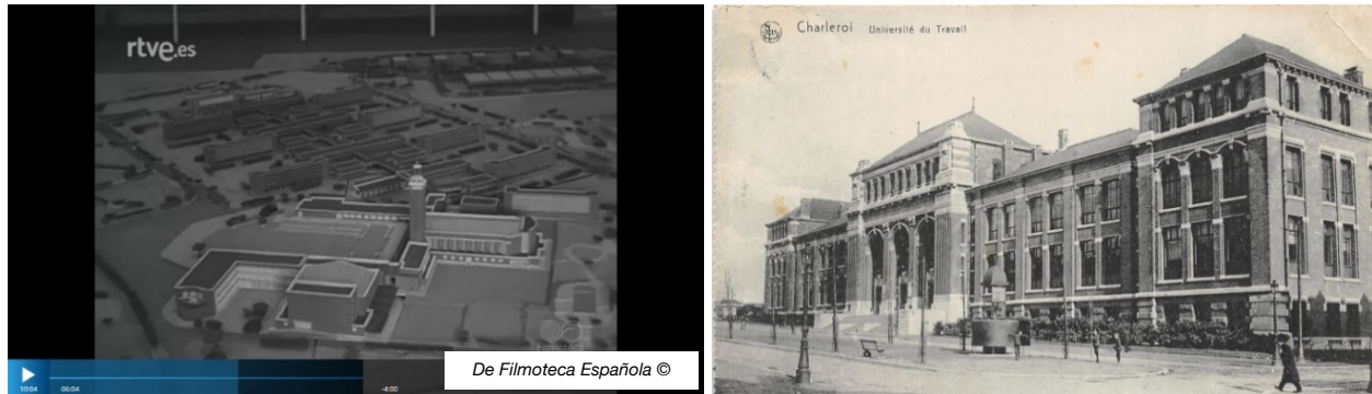
Image 3: Model of the José Antonio Primo de Rivera Labor University (Seville) and main facade of the Belgian UT. Source: Noticiario n. ° 695A (30/04/1956) and Postcard retrieved from https://www.geneanet.org/cartes-postales/view/7696651#0 .
