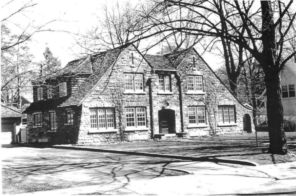
Figure 7: This Tudor-style Arts & Crafts cottage at 9 Brant Road South was built in 1929. It is constructed of mauve sandstone and has a cedar shingle roof. Photo: John S. Hagopian, 1998.
