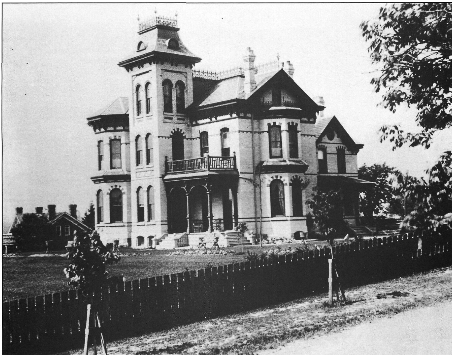
Figure 6: Paris postmaster and militaryman Captain Cox built this luxury home on a large Quality Hill lot bordered by Boardway Street East, Banfield Street, and Grand River Street North During 1885-1886, just after the completion of the waterworks in 1884. The water main which served this property ran north along Broadway Street East to Banfield Street, where it branched west to the railroad 'Junction'. The mansions of Charles Whitlaw (across Banfield) and John Penman (across Grand River Street North) abutted this property. William Kipp, Sr., Private collection.
