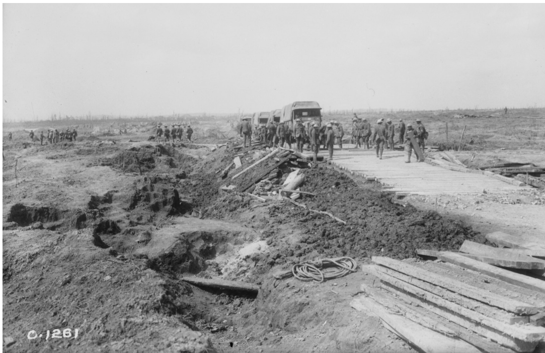
Figure 5. Laying a road over the crest of Vimy Ridge. April, 1917. Source: PA-001226, box number: 83,7435, 15, O-1261, Library and Archives Canada.
