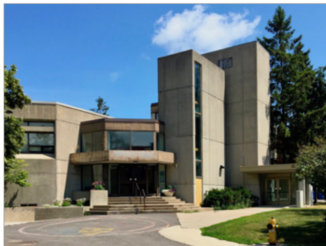
FIG. 16. MAIN ENTRANCE, HARRISON-LECAINE HALL (R.J. THOM ARCHITECTS, 1972-1974), QUEEN'S UNIVERSITY, KINGSTON. | JAMES ASHBY, 2019.
