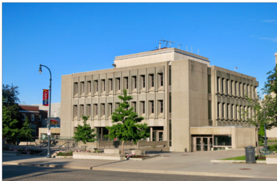
FIG. 5. JEFFERY HALL (MARSHALL & MERRETT; STAHL, ELLIOT & MILL, 1969), UNIVERSITY AVENUE, QUEEN'S UNIVERSITY, KINGSTON. | JAMES ASHBY, 2019.
