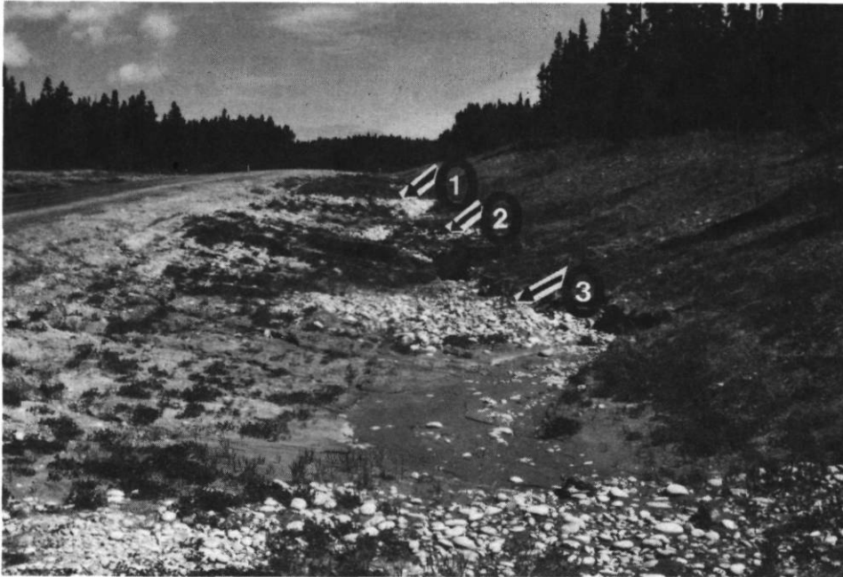
FIGURE 2. Section of road ditch mapped in Figure 1. Numbers identify gravel pads.
