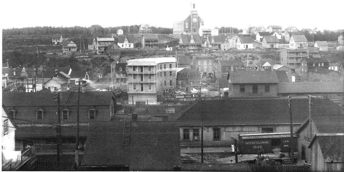
Rivière-du-Loup Station After the Turn of the Century. Church of Saint-Ludger in Background
