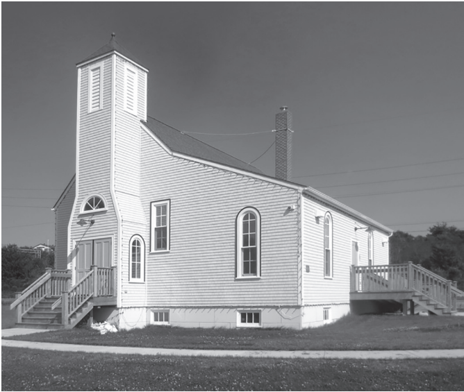
Figure 5. Rebuilt Africville Church. Photograph by V. Prouse.
