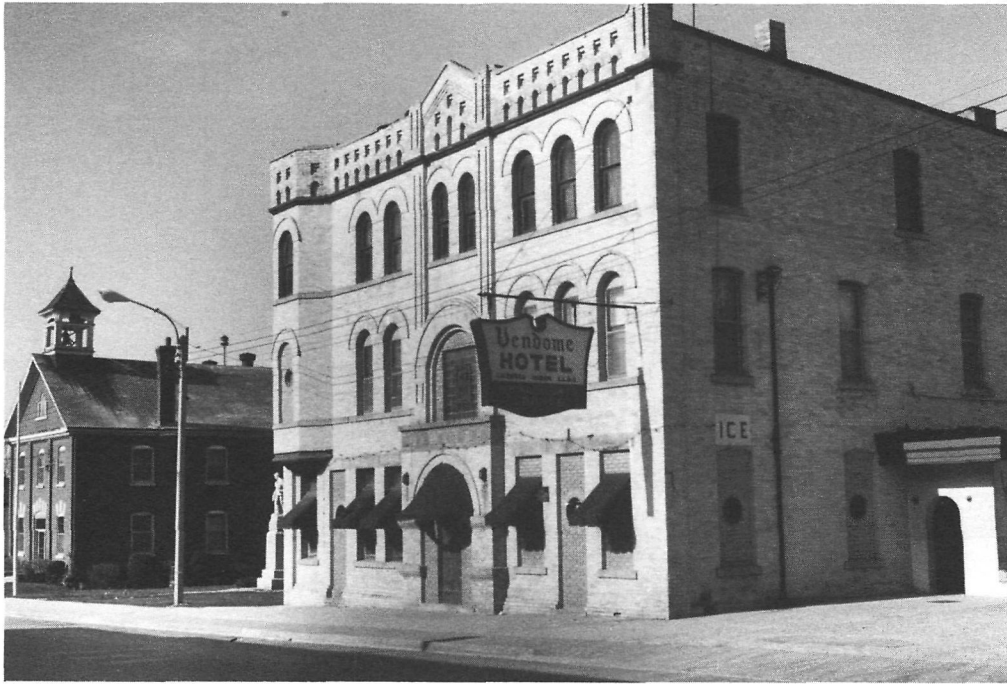
FIGURE 12. Restored hotel on the main street of Teeswater.
