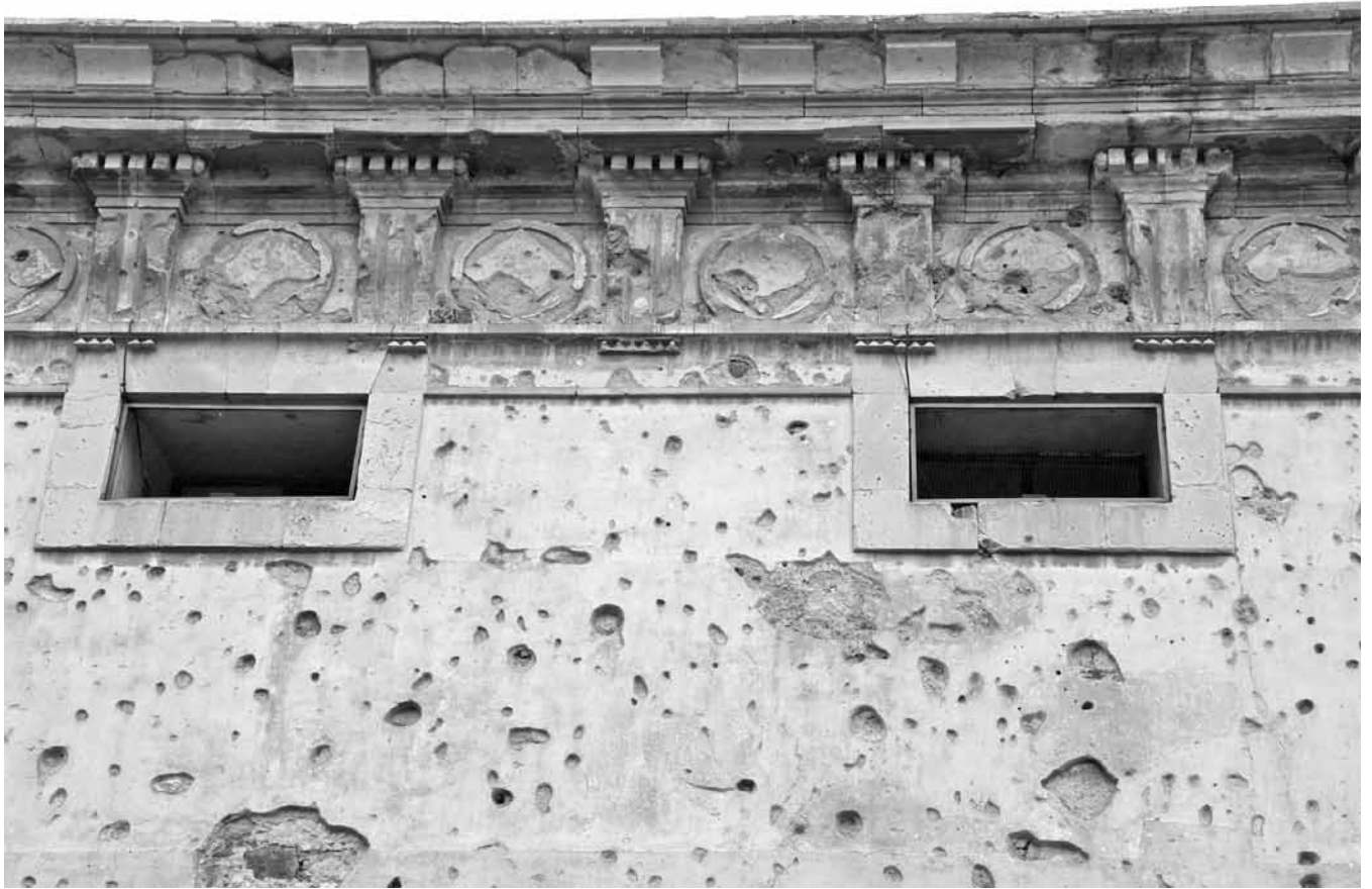
Figure 9. Granary of Granaditas, Guanajuato. Cornice with triglyphs and metopes crowning the façades (Photo: author).
