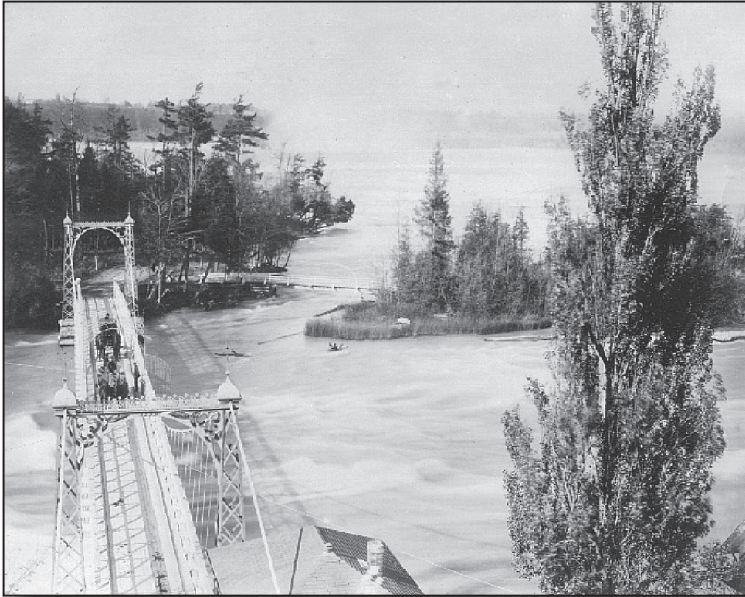
The toll bridge to Sutherland Macklem's island attractions in 1880. (Niagara Falls Public Library)
