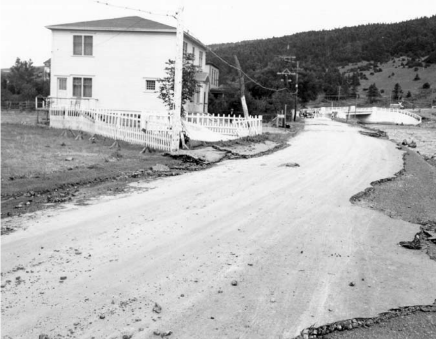
Figure 4. Flood damage on Southside Road, September 1948 (St. John's City Archives, used with permission).
