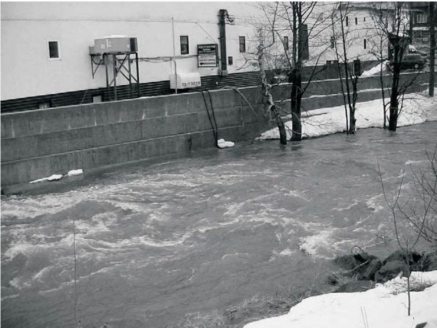
Figure 12. Flood protection, Waterford River, constructed after 2001 flood.
