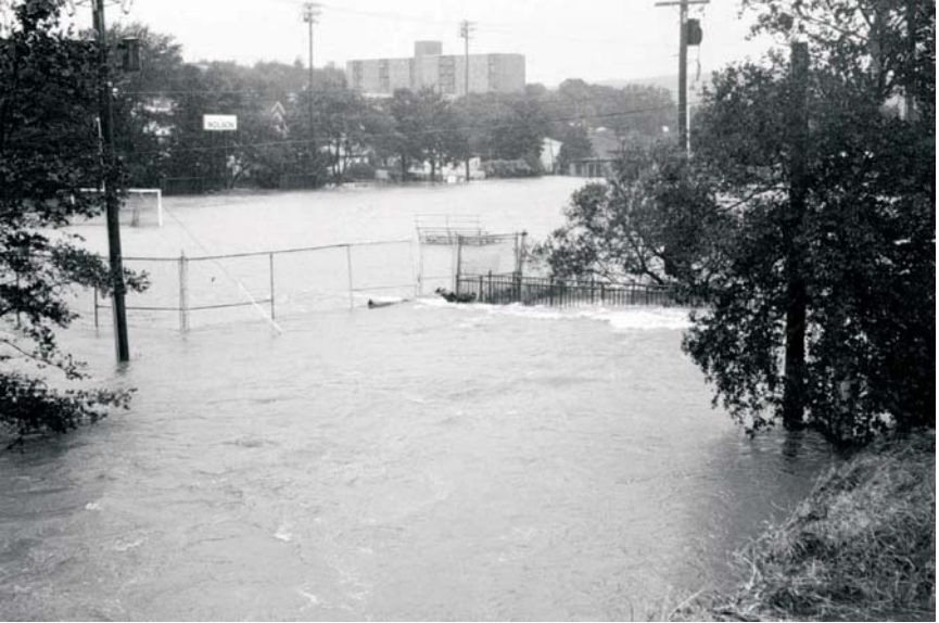
Figure 10. Floods cover soccer field at head of Quidi Vidi Lake, September 2001. Note footbridge over Rennie's River forming dam as it blocks flood waters.
