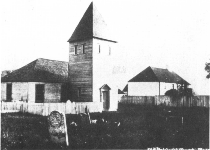
Pl. 1A: Anglican church (1787), cemetery and the courthouse at Placentia. The church and cemetery are on the same site as the French church, established by the Recollects in 1689, and used by the English after 1713.
