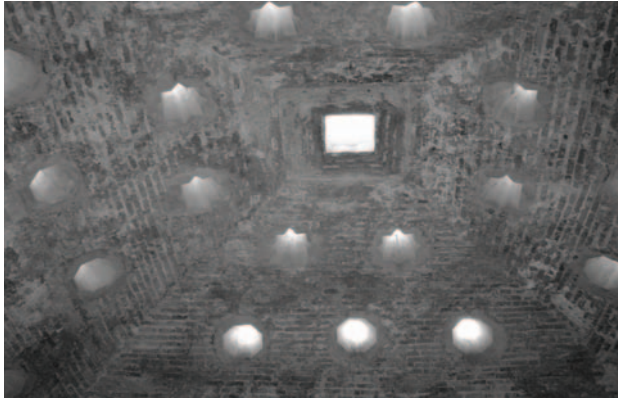
Picture 3 – A bottle glass domed structure
