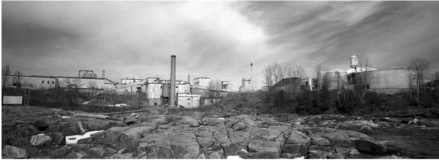
The Sturgeon Falls paper mill shortly before its demolition.
