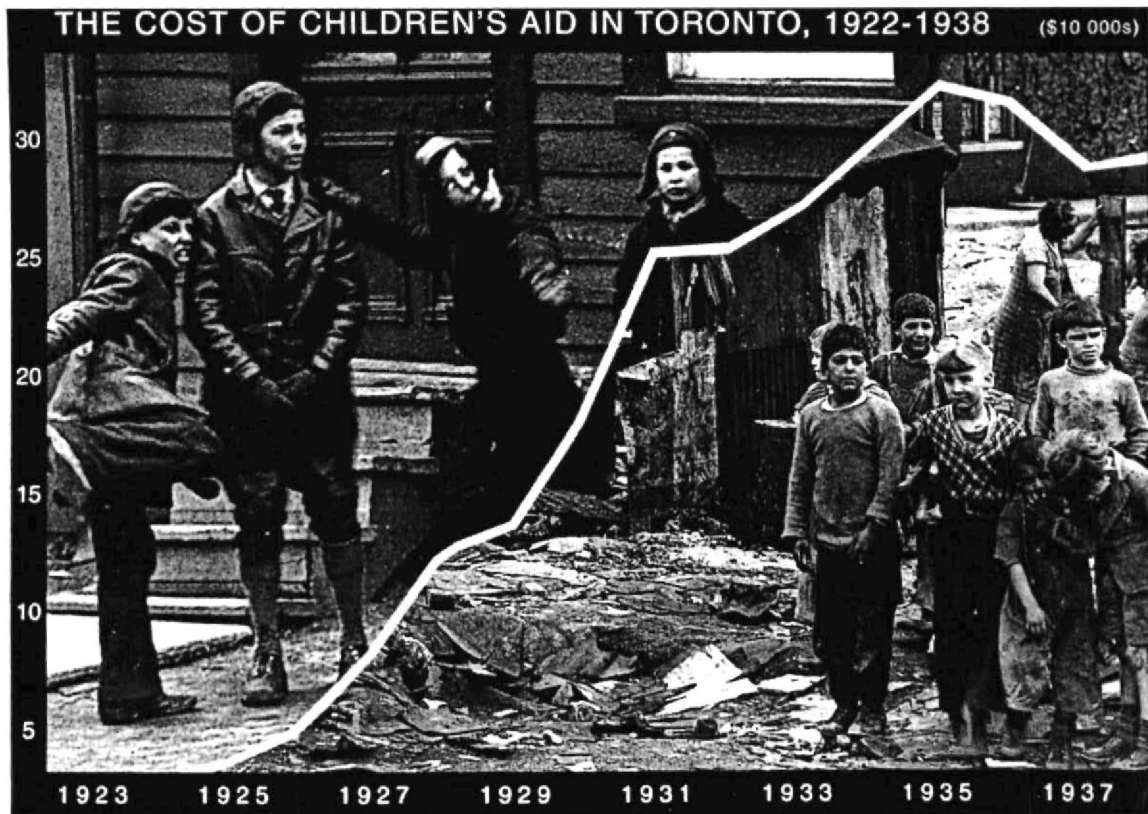
Left: City of Toronto Archives, Department of Public Works and Housing, 33-290. Right: City of Toronto Archives, Department of Public Works and Housing, 33-231. Design: Marcus Klee.
