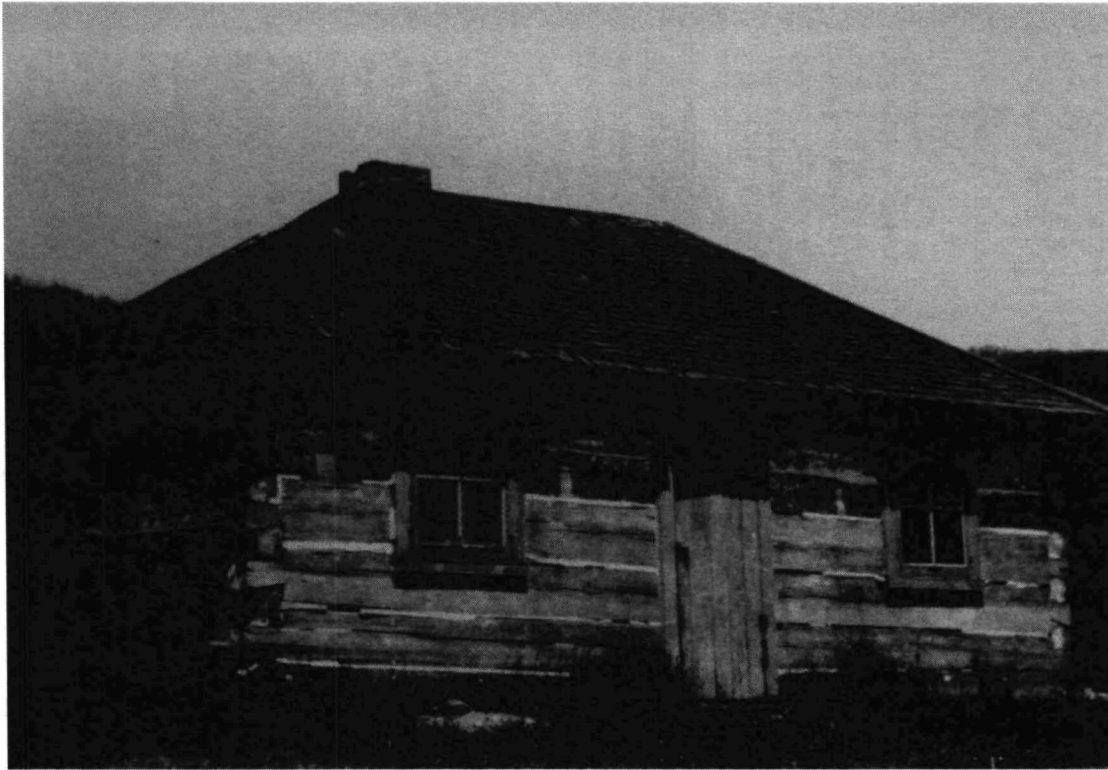
Fig. 4. Fort Wellington guard house where soldiers were held prisoner for drunkenness, fighting, and other misdemeanors. The building has been demolished. Historical photograph provided by Dennis Carter-Edwards, Parks Canada.
