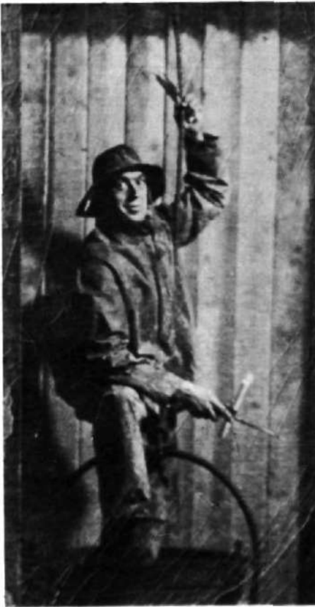
The miner, dressed in wet clothes, is about to descend into the shaft perched on an ore bucket. Note the candle in one hand and the dynamite in the other. The photograph was taken from a postcard written in 1907. (In author's possession).
