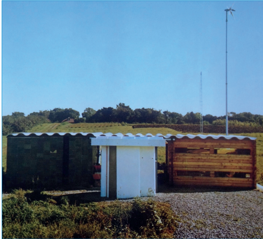
FIG. 7. MCHG, ECOL , 1972, SAINTE-ANNE-DE-BELLEVUE, QUEBEC, CANADA, FROM THE ECOL OPERATION: ECOLOGY + BUILDING + COMMON SENSE (MCHG, DECEMBER 1972, COVER PAGE). COURTESY OF VIKRAM BHATT ON BEHALF OF THE MCGILL UNIVERSITY MINIMUM COST HOUSING GROUP.
