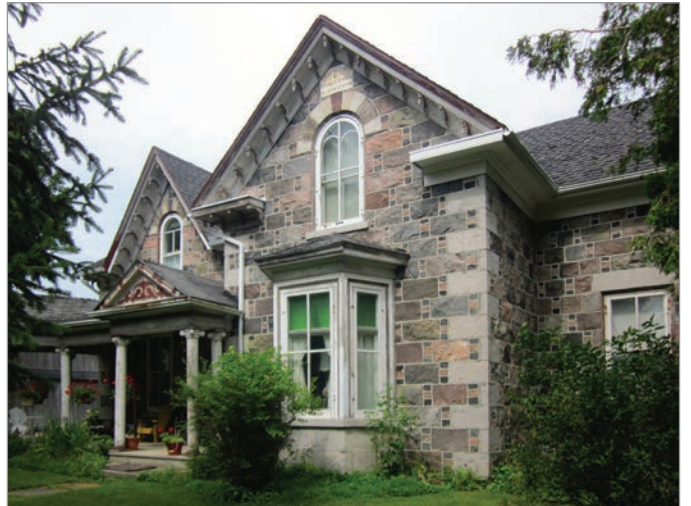
FIG. 13. SEATON HOUSE, 25TH LINE, NO. 6594, LAKESIDE, OXFORD COUNTY. | KAREN E. ARMSTRONG.
