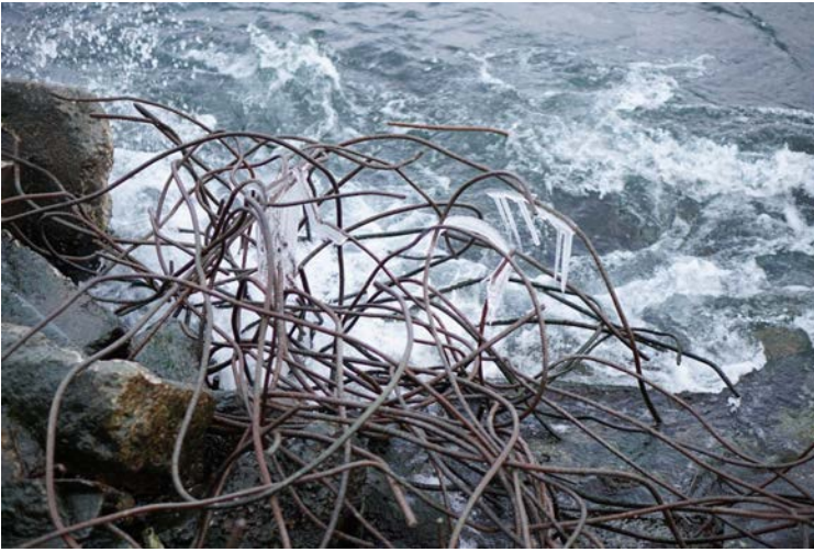
Figure 8: Rebar at Tommy Thompson Park
