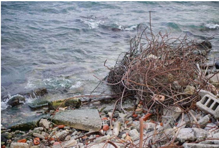
Figure 7: Rebar at Tommy Thompson Park
