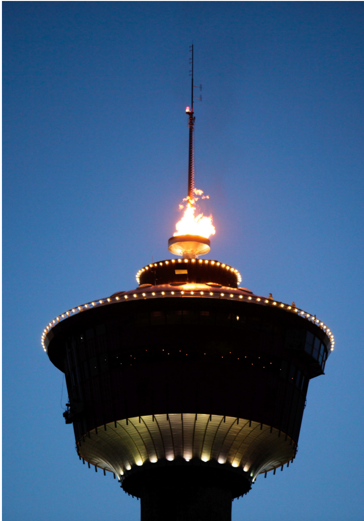
Figure 6: cauldron atop the Calgary Tower during the Vancouver Olympic Games, 18 January 2010
